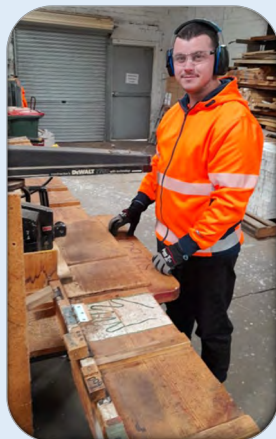
Tom preparing to cut the wood to length.
